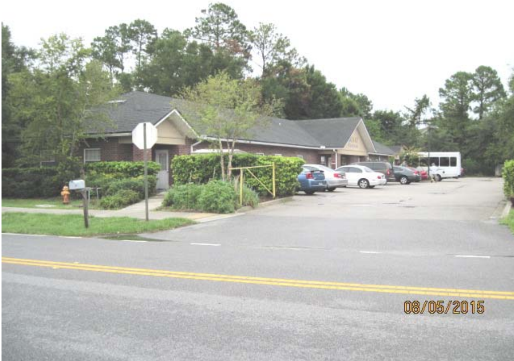
Existing commercial office across Cortez Road
